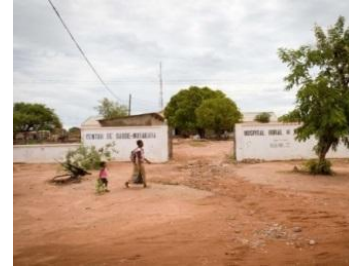
Figura 37 – Hospital Rural de Mutarara
